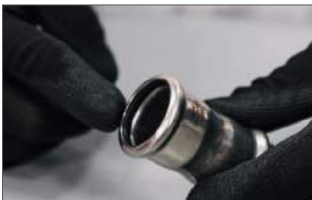
Controllo O-ring / Checking the sealing ring
